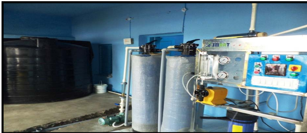
RO Water Plant Provided in Srinagar village
