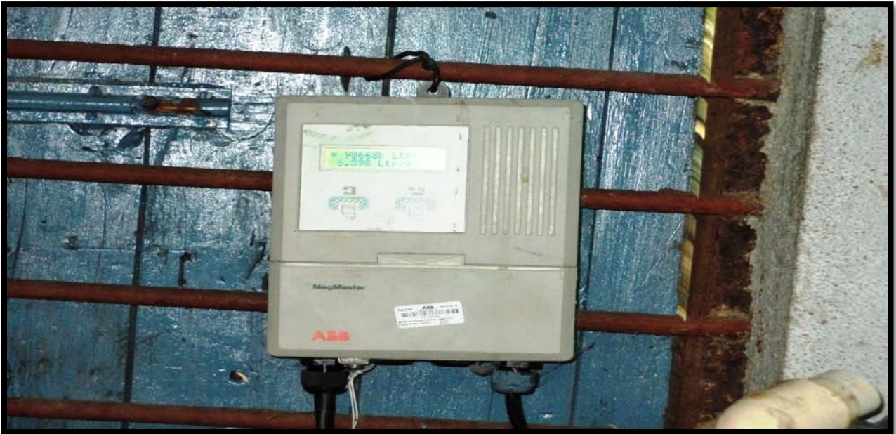
Domestic water meter
